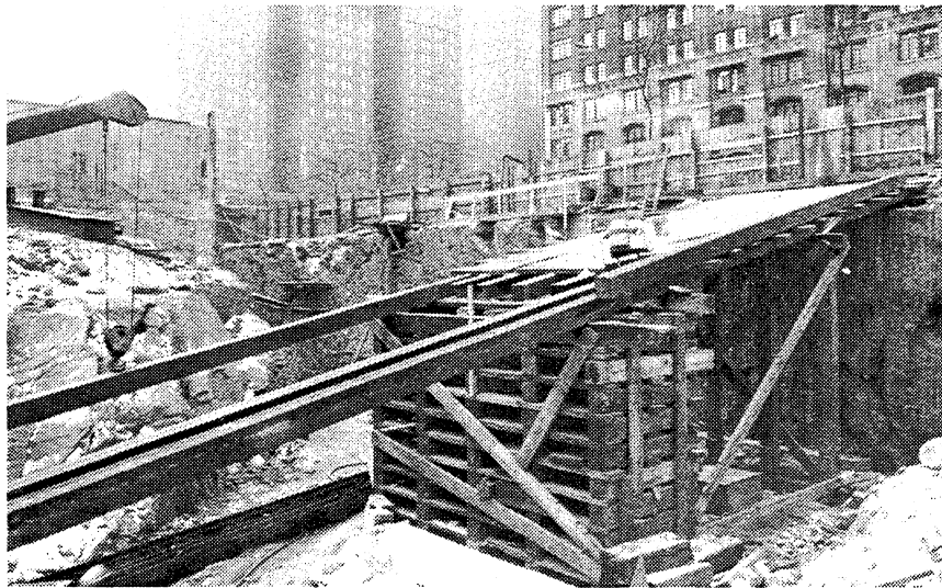
Fig. 6-1 Construction ramps are usually fabricated using a combination of steel and timber
