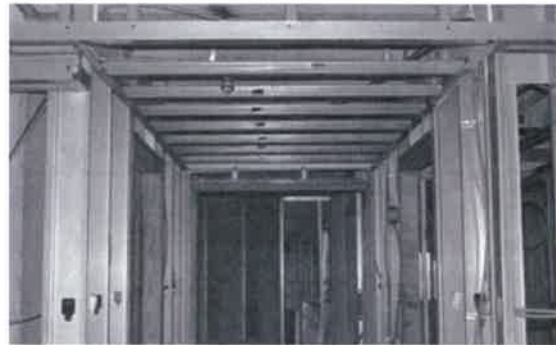
Corridor framing using traditional steel studs
