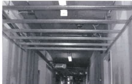
ShortSpan Framing and Locking Angle Molding make drywall framing faster and easier
