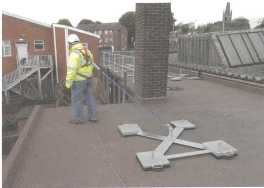
FIGURE 9 Fall restraint system
