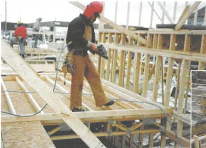
Unprotected stairwell
