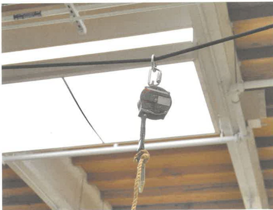
FIGURE 43 Horizontal lifeline deflection
