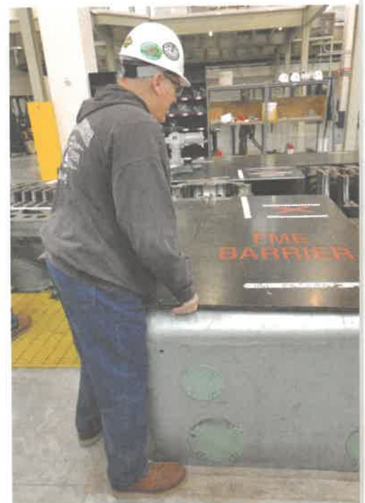
FIGURE 10 Placing an FME cover
