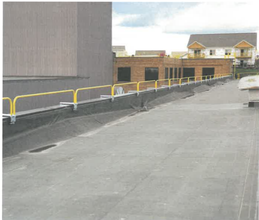
FIGURE 14 Parapet wall midrail
