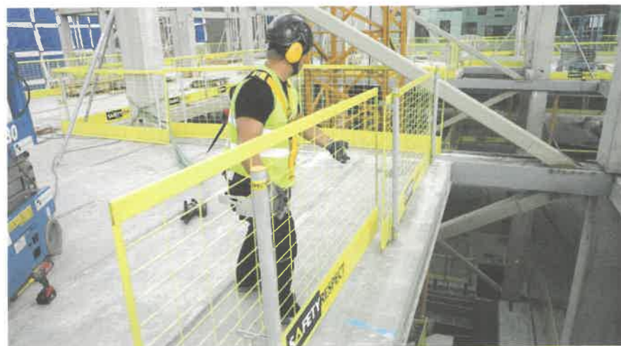
FIGURE 23 Guardrail with removable section
