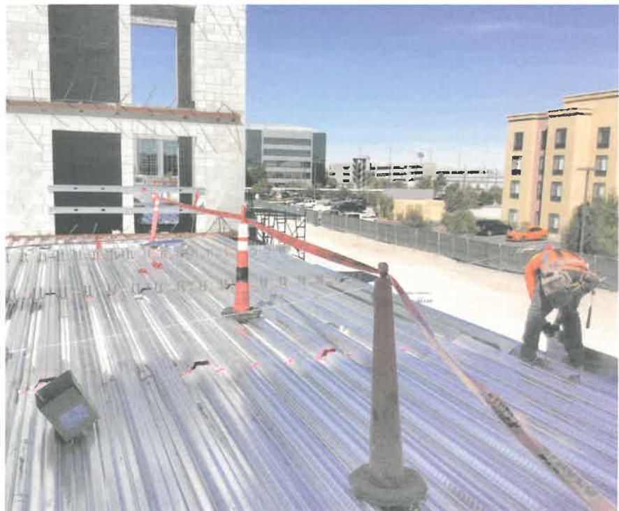
FIGURE 8 Controlled decking zone (CDZ)
