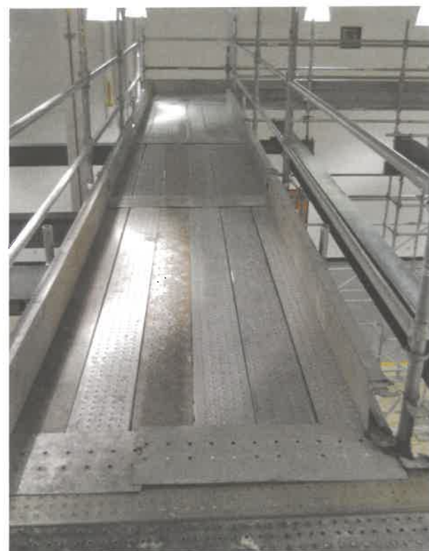
FIGURE 8 Guardrail system with toeboards
