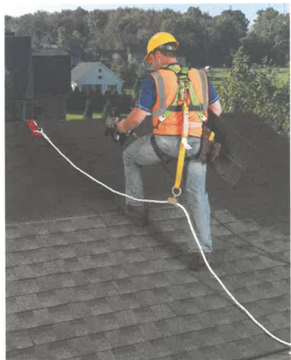
FIGURE 40 Using a vertical lifeline with a rope grab
