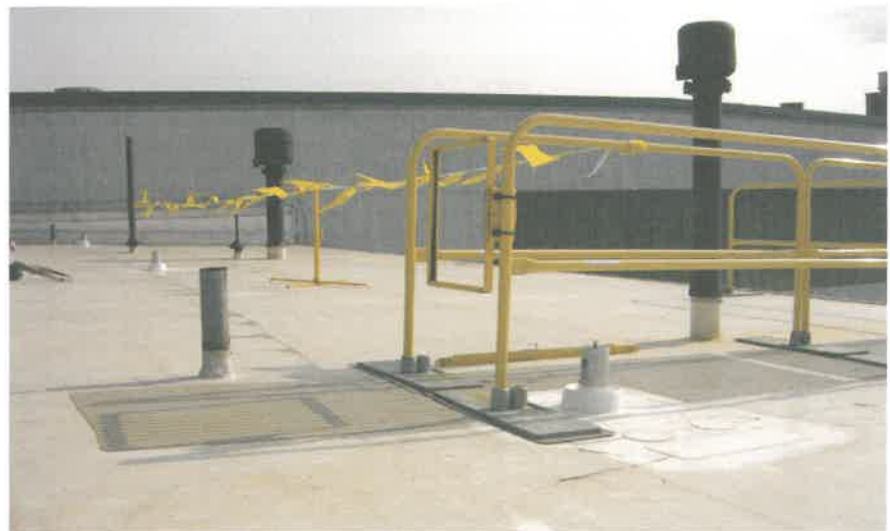
FIGURE 6 Warning line access path
