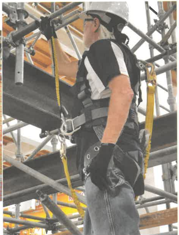
FIGURE 59 Active fall protection
