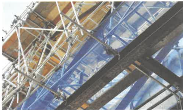
FIGURE 32 Scaffold safety net
