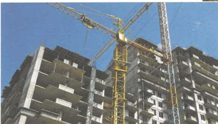
Unprotected leading edge
