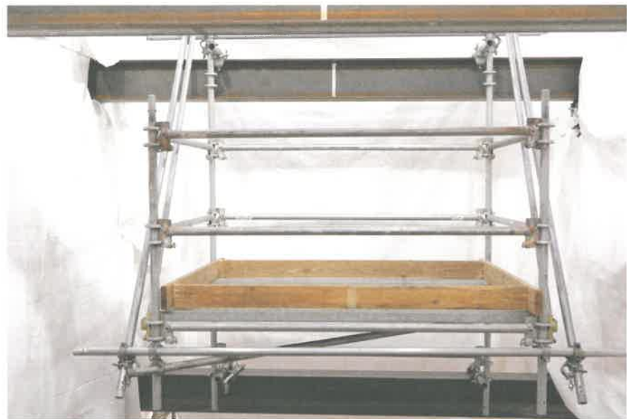
FIGURE 4 Toeboards and guardrails
