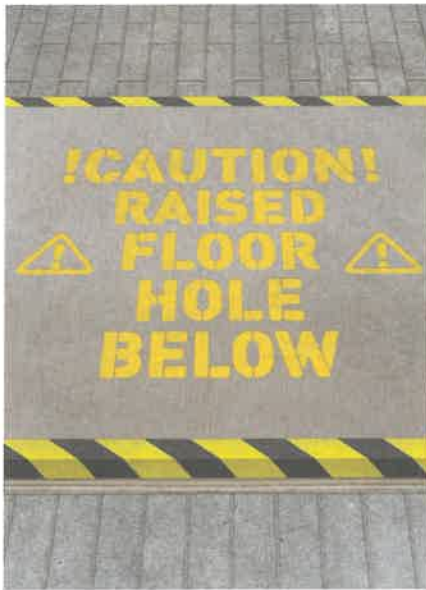
Typical plywood hole cover
