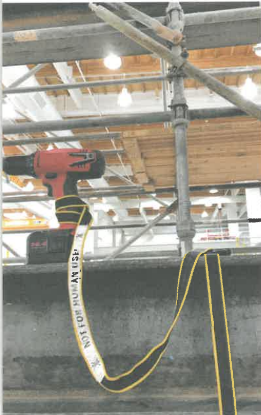
FIGURE 22 Drill anchored to a structure
