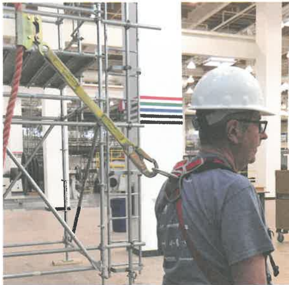
FIGURE 4 Vertical lifeline attached to a D-ring
