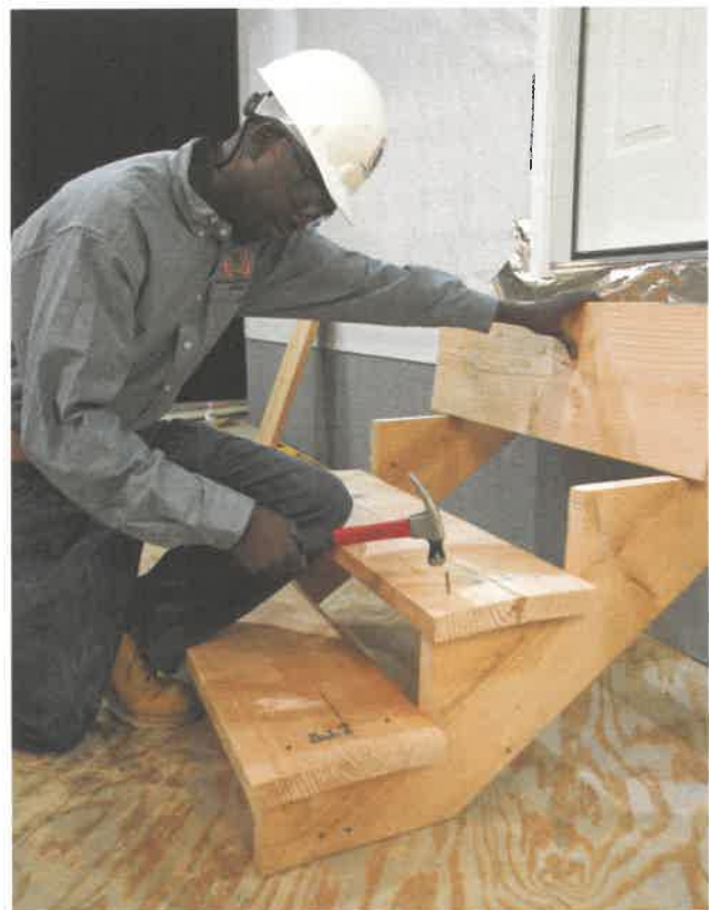
FIGURE 47 Building temporary stairs
