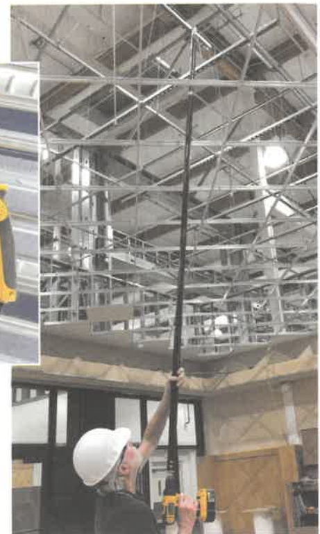
FIGURE 6 Fastening ceiling wire using a tool extension
