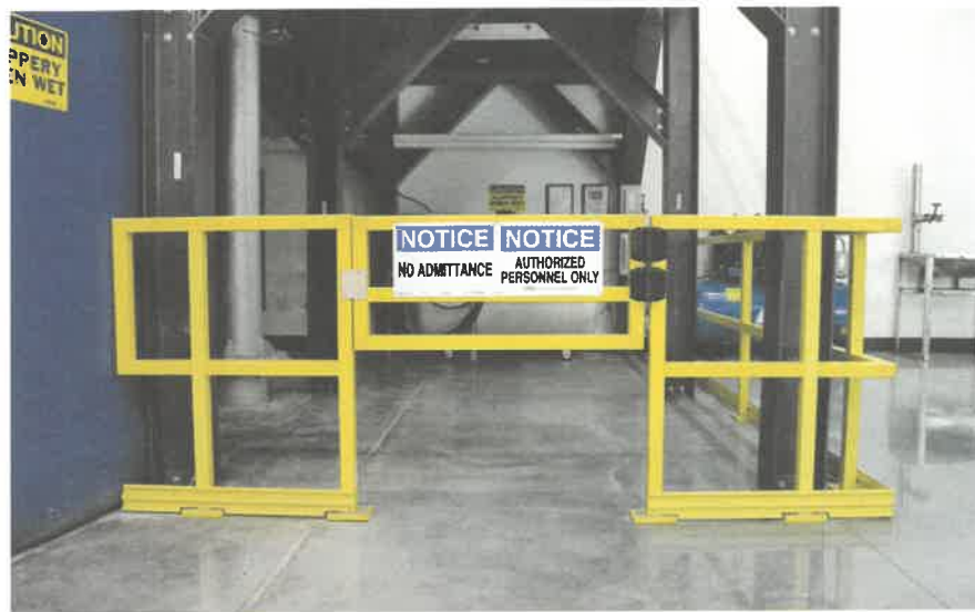
FIGURE 22 Guardrail with gate access
