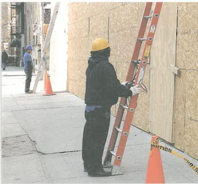
FIGURE 12 Proper ladder setup
