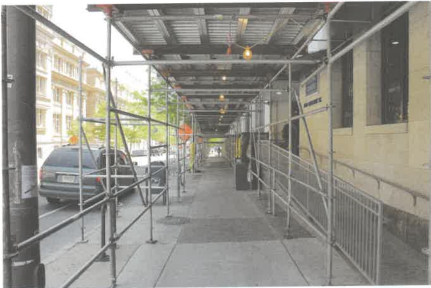
FIGURE 9 Lighted pedestrian passageway
