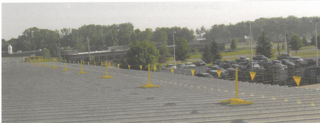
FIGURE 1 Warning line system
