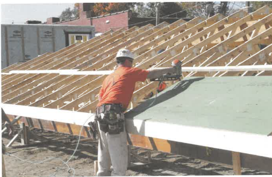
FIGURE 2 Framing a roof section
