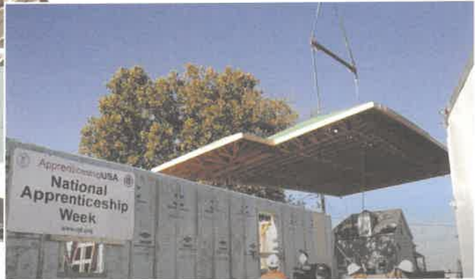
FIGURE 4 Placing the roof section
