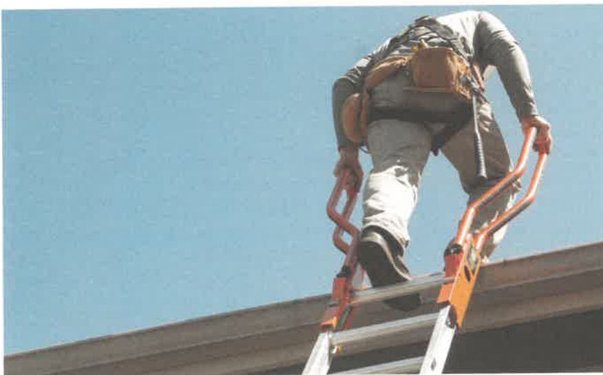
FIGURE 32 Ladder with walk-through extensions
