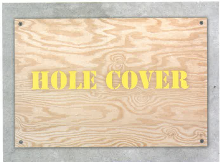
FIGURE 38 Marked hole cover
