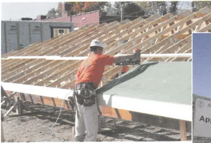
FIGURE 3 Framing a roof section
