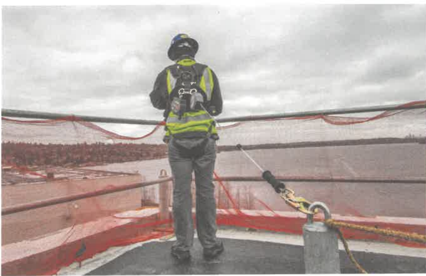
FIGURE 38 SRL-LE anchored at foot level
