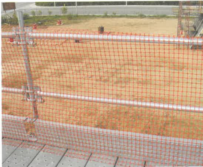
FIGURE 58 Toeboards and mesh netting
