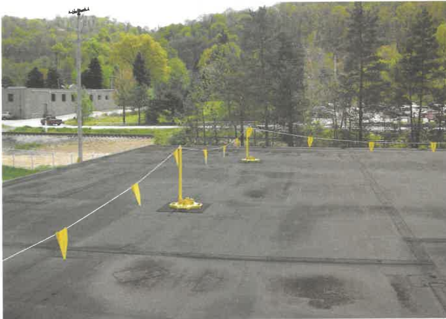
FIGURE 4 Warning line system
