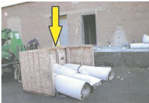
Three-sided skip box used to elevate carpet rolls to window
