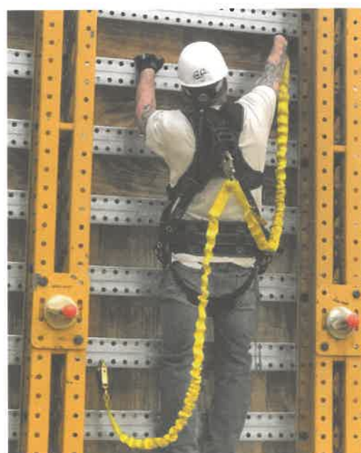
FIGURE 31 Using a twin-legged lanyard
