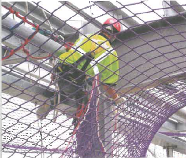
FIGURE 34 Inspecting safety nets
