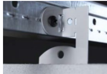
Figure 46 - Screw Attached Embedded Clip
