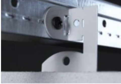
Figure 57- Attached Anchor Clip
