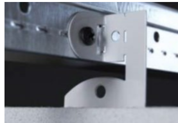
Figure 46 - Screw Attached Embedded Clip
