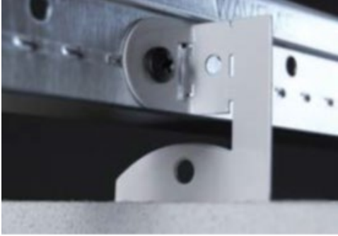
Figure 57- Attached Anchor Clip
