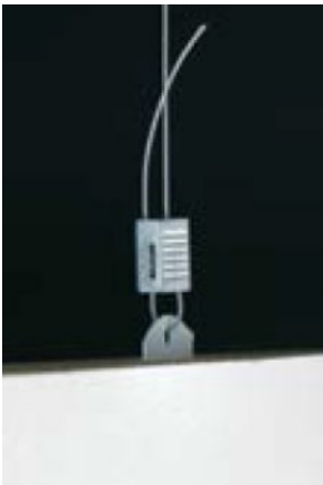
Figure 45 - Embedded Clip
