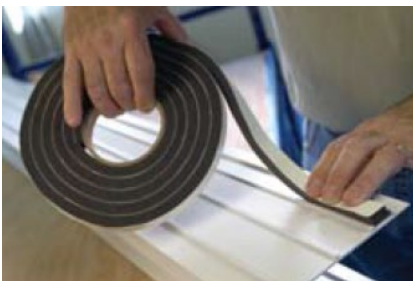
Figure 12 - Installing Foam Gasket
