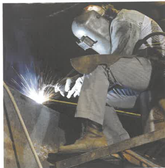
FIGURE 1 Welder wearing proper clothing
