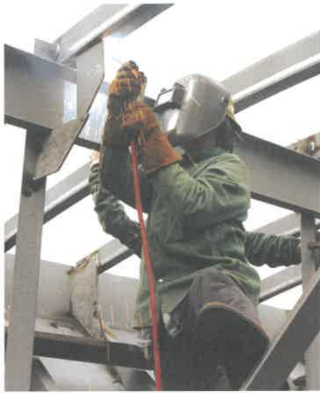
FIGURE 3 Welding with SMAW
